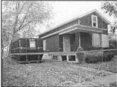
House on Oxford Street undergoing asbestos removal
