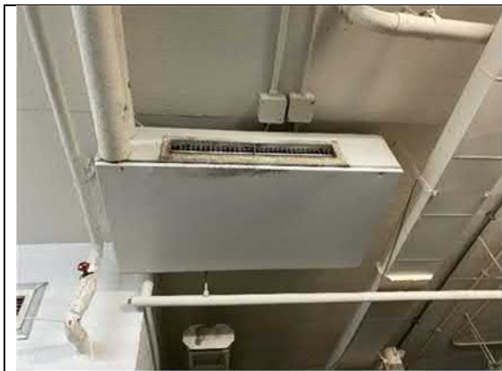
Typical Fan Coil Unit
