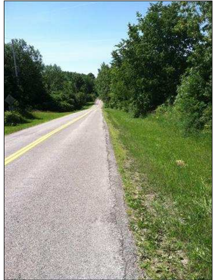
Photograph 22. Brew Road, looking south.
